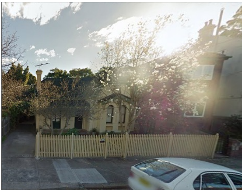
Figure 39: No. 63 Morris Street, Summer Hill. Locally listed item. Google Maps, 2016.
