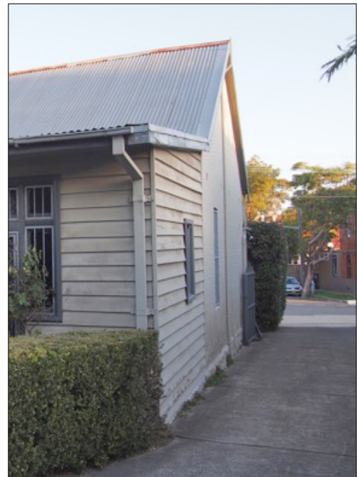
Figure 13: Western elevation of the dwelling, looking south.
