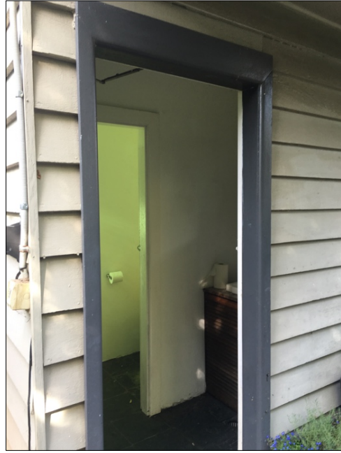
Figure 27: Fibro lining and external bathroom fit out.
