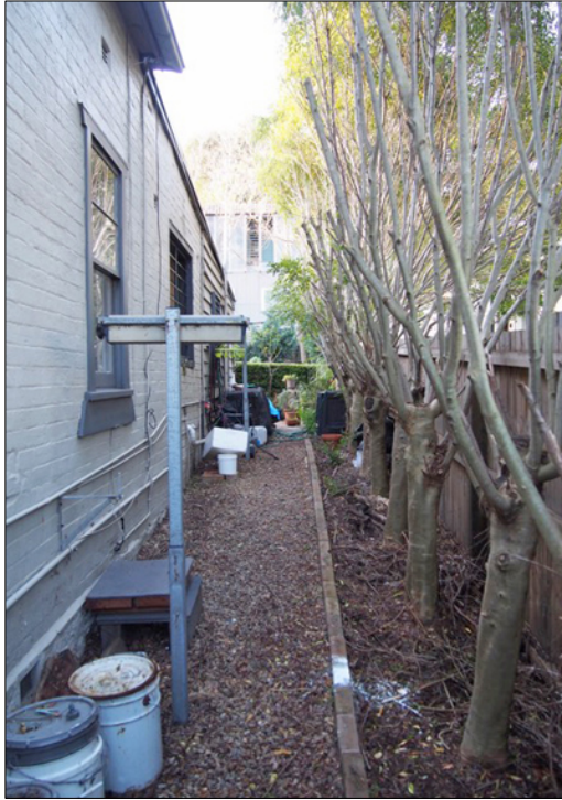
Figure 10: The eastern side of the dwelling, looking north along the principal building form.
